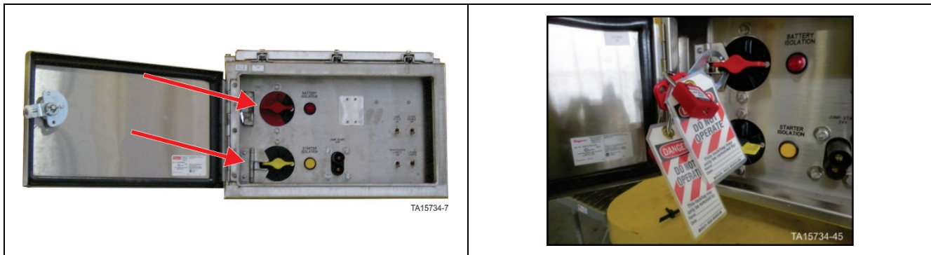
Figure 7. Battery Isolation Box – Battery isolation switch in OFF position with locks in place
